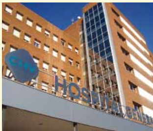
Hospital General de Vic
